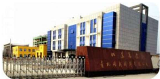
Shandong Wanda Orgonosilicon New Materials (Plant)
